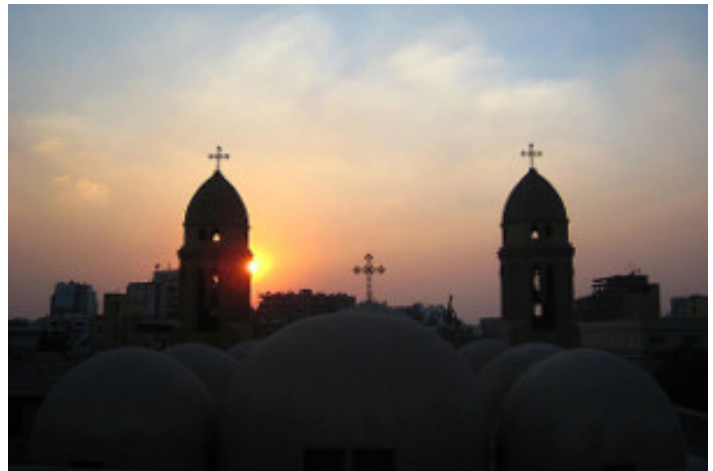
A Coptic church building in Egypt. Photo: Flickr / Andrew A. Shenouda ( CC )
